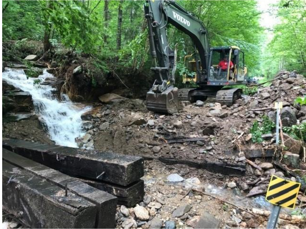
Repair and construction on Presidential Rail Trail
